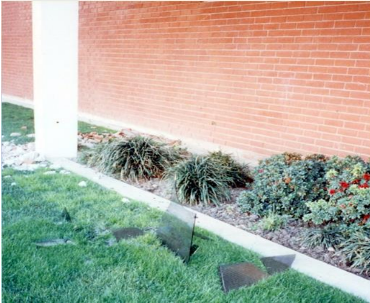
Figure 2.4.1-2 Shards of broken untempered glass that fell several stories from a multistory building in the 1994 Northridge Earthquake. Failures of this type can be very hazardous, especially if glazing is located above exit ways (FEMA 74, 1994).
