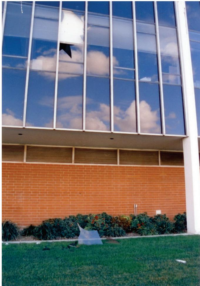
Figure 6.3.1.4-1      Shard of broken untempered glass that fell several stories from a multistory building in the 1994 Northridge Earthquake (Photo courtesy of Wiss, Jenney, Elstner Associates).
