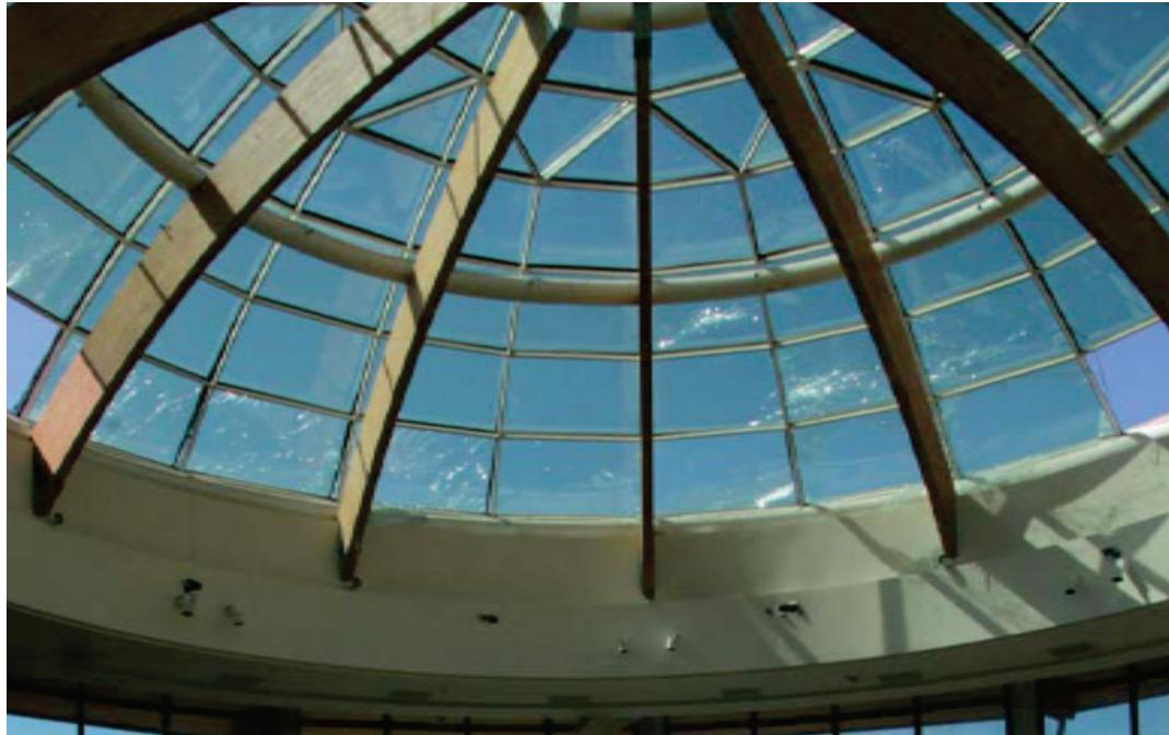
Figure 6.3.1.4-5 Overhead glazing damage from the 2010 Chile Earthquake (Photo courtesy of Eduardo Miranda, Stanford University).
