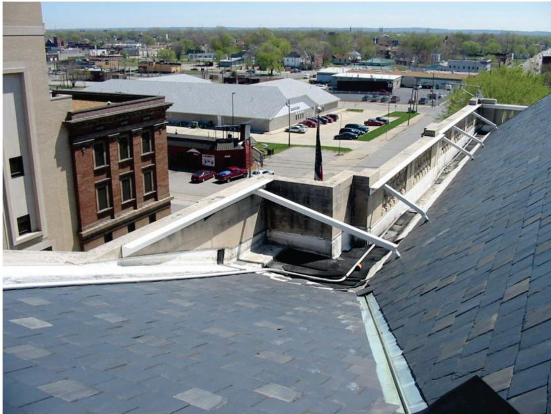
Figure 6.3.5.1-5 Bracing of unreinforced masonry parapet (Photo courtesy of Degenkolb Engineers).
