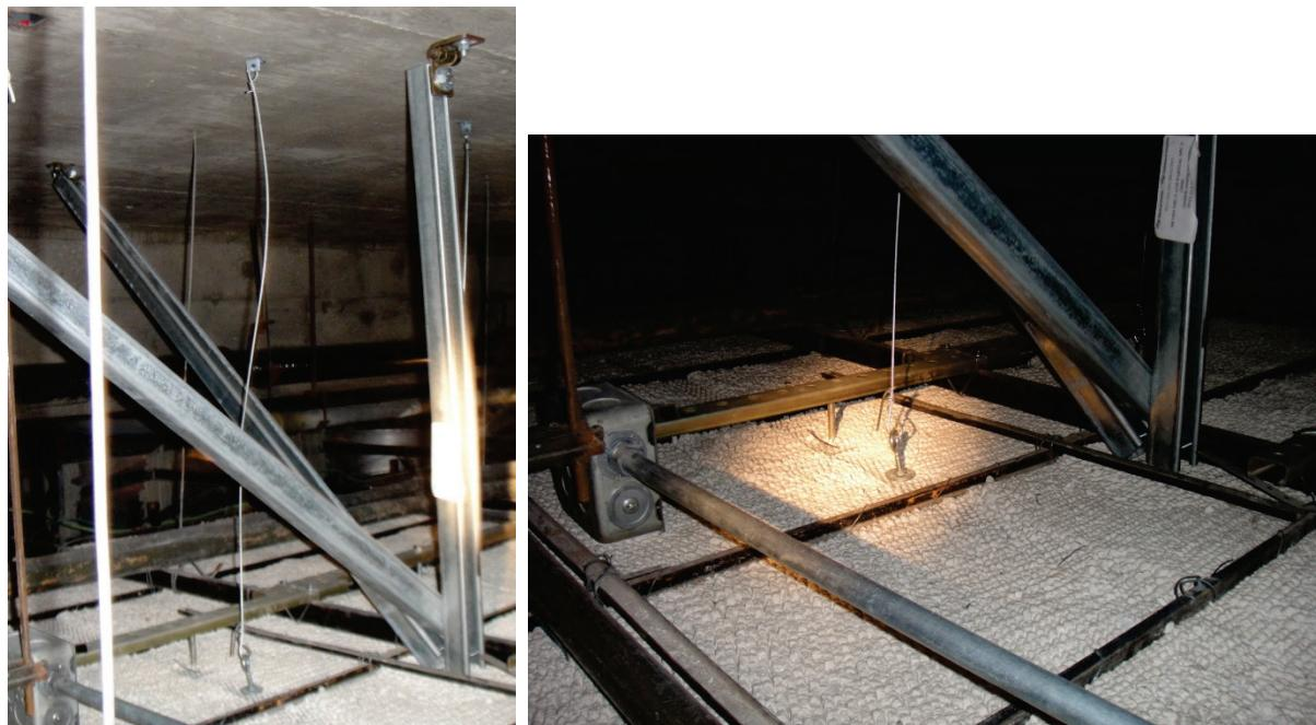
Figure 6.4.9.2-3      Independent vertical support for surface-mounted light fixture in suspended gypsum board ceiling located in California hospital. Eye hook and slack wire from fixture is tied to concrete slab above. The rigid bracing in the photos is attached to the ceiling grid, not the light fixture (Photos courtesy of Maryann Phipps, Estructure).
