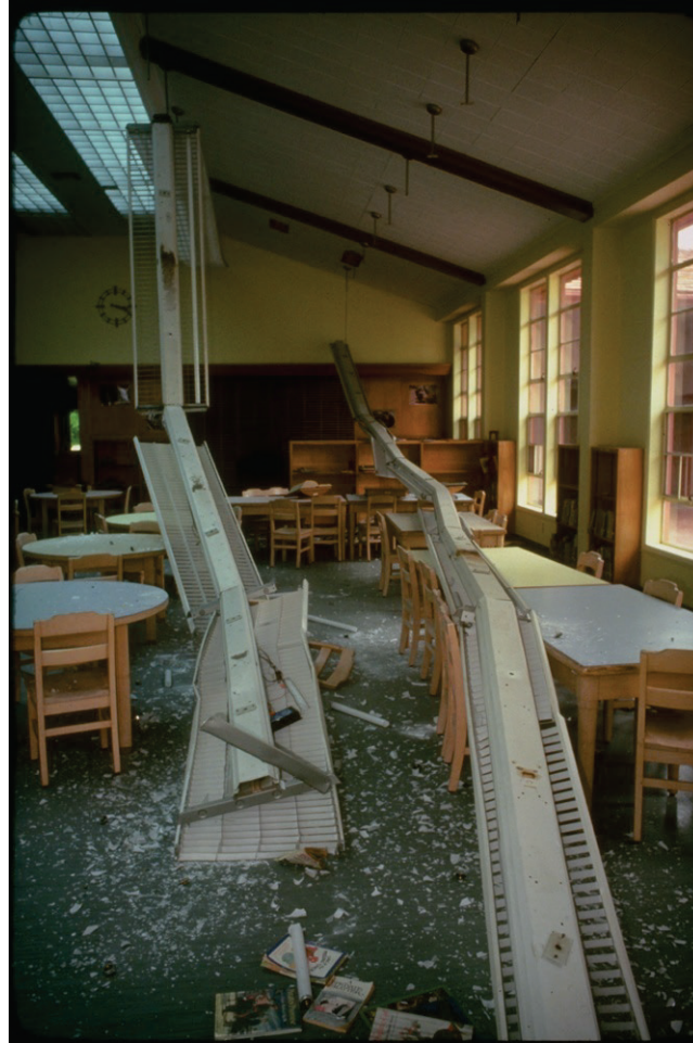
Figure 6.4.9.3-2 Failure of pendant light fixtures at Northridge Junior High School as a result of the 1994 Northridge Earthquake. In this example, the support stem failed at the fixture connection and the stem is still attached at the ceiling (Photo courtesy of Gary L. McGavin).
