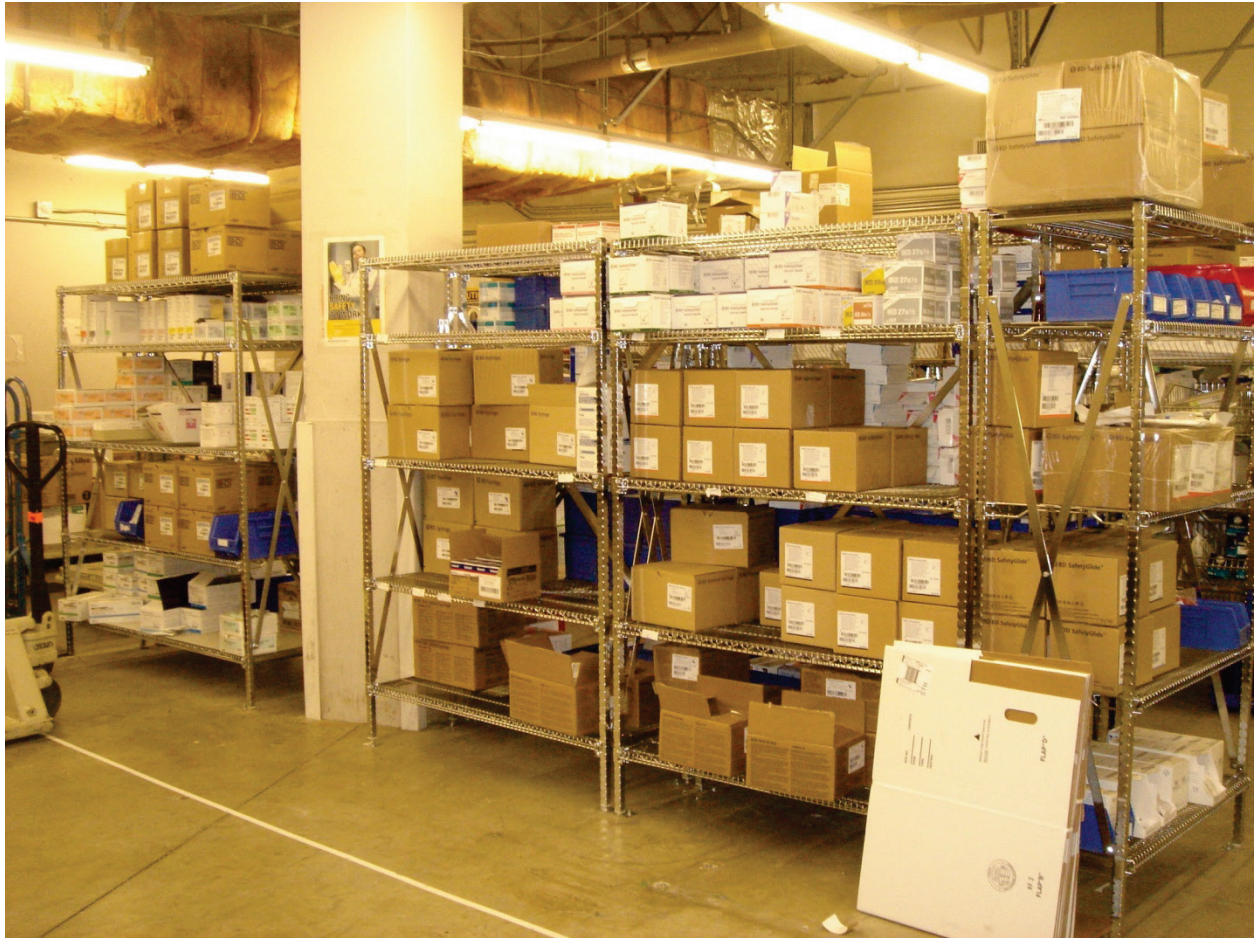
Figure 6.5.1.1-7 Fixed base shelving units anchored directly to concrete slab through base plate (Photo courtesy of Maryann Phipps, Estructure).
