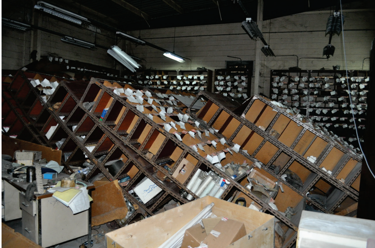
Figure 6.5.1.1-1 Collapse of row of unanchored freestanding shelving units containing spare parts at an electric power plant in Port-au-Prince in the 2010 magnitude-7 Haiti Earthquake (Photo courtesy of Eduardo Fierro, BFP Engineers).
