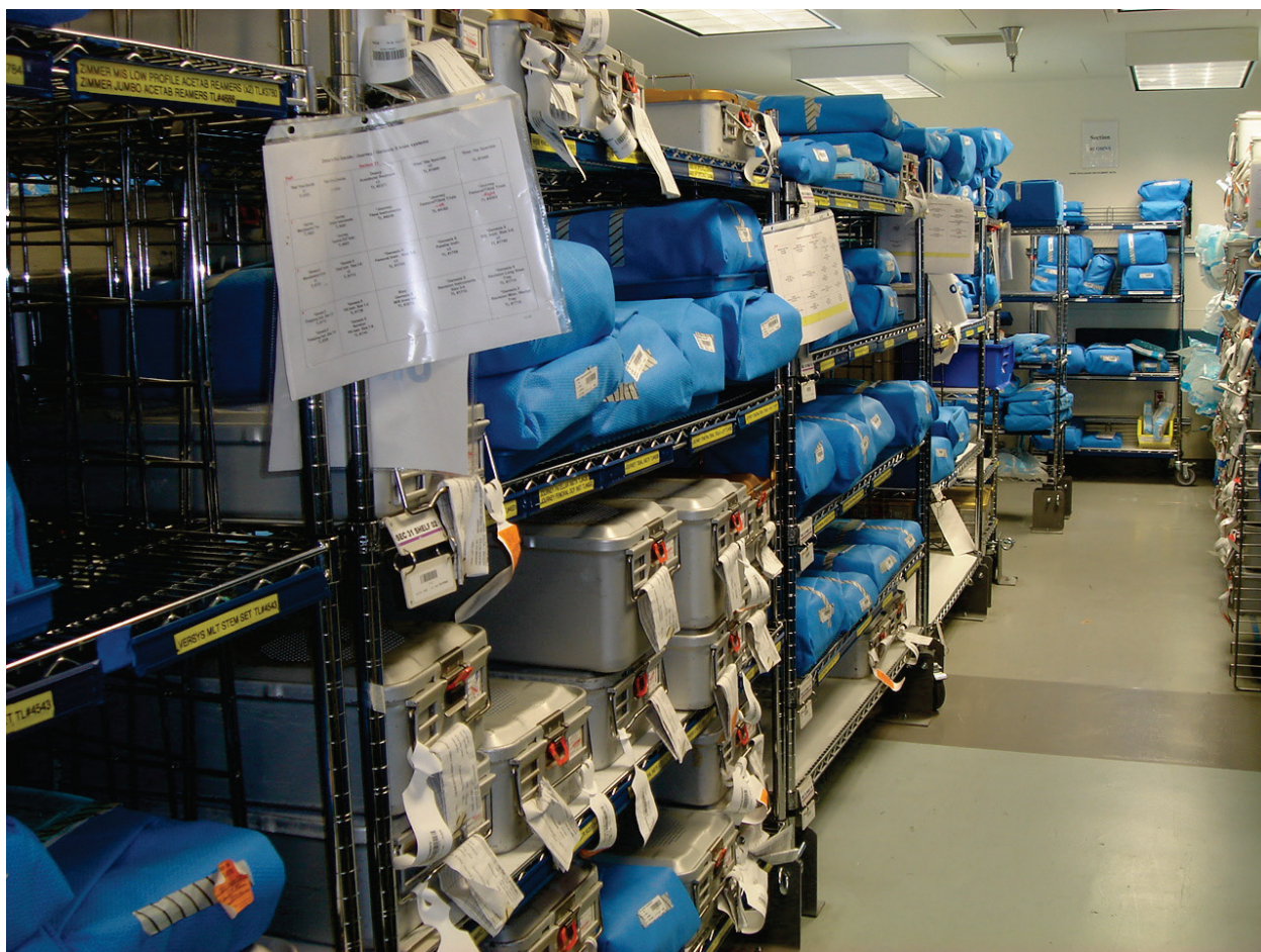
Figure 6.5.1.1-3 Mobile carts restrained at base with clip angles anchored to the floor and removable eyebolts attached from each cart to the angles (Photo courtesy of Maryann Phipps, Estructure).
