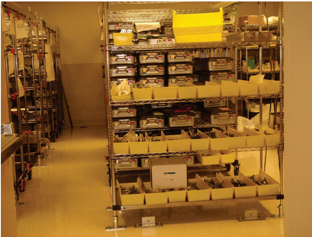
Figure 6.5.1.1-5 Fixed base shelving units anchored with optional seismic base plate offered by manufacturer (Photo courtesy of Maryann Phipps, Estructure).
