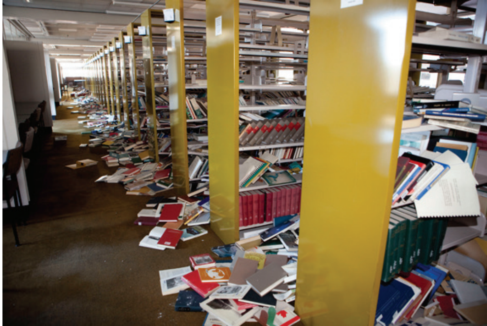
Figure 6.5.2.2-4 Shelving units with longitudinal ties did not fall over but all of the contents spilled to the floor in the 2010 Canterbury Earthquake. The use of lips or wires would have prevented the damage.(Photo courtesy of University of Canterbury).
