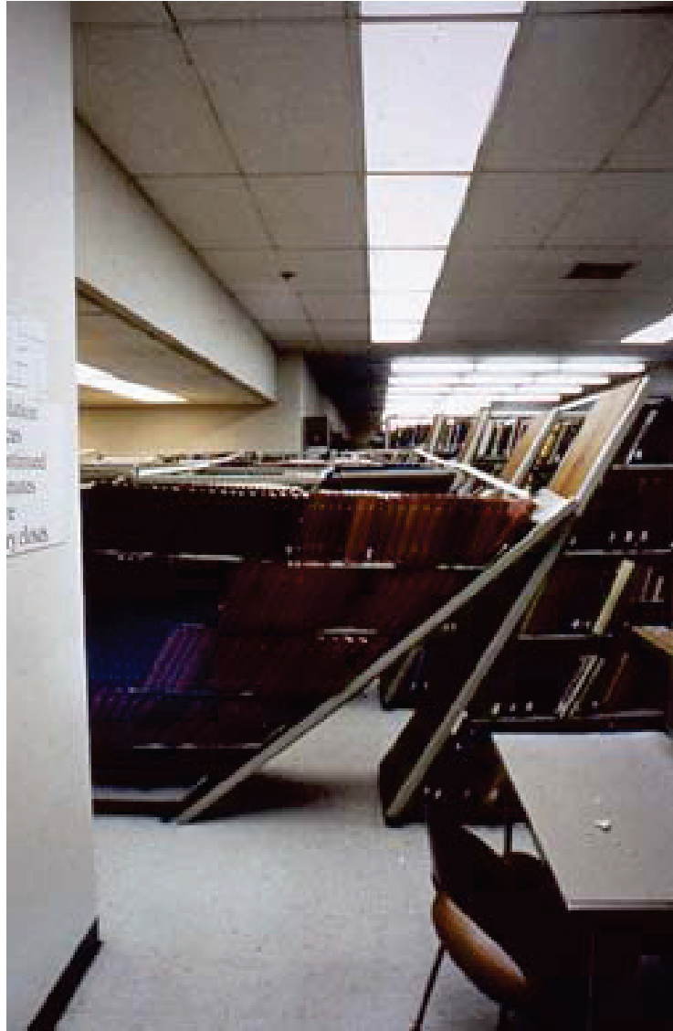
Figure 6.5.2.2-3 Longitudinal failure of library shelving units (Photo courtesy of NISEE-PEER, U.C. Berkeley). Transverse ties used to tie units together but this was not enough to prevent longitudinal failure.
