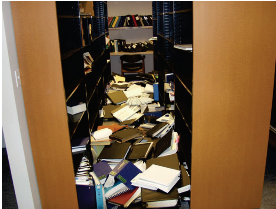
Figure 6.5.2.2-5 These shelving units remained in place but all of the contents spilled in the 2010 magnitude-6.5 Eureka, California Earthquake (Photo courtesy of Steve Mahin, PEER).
