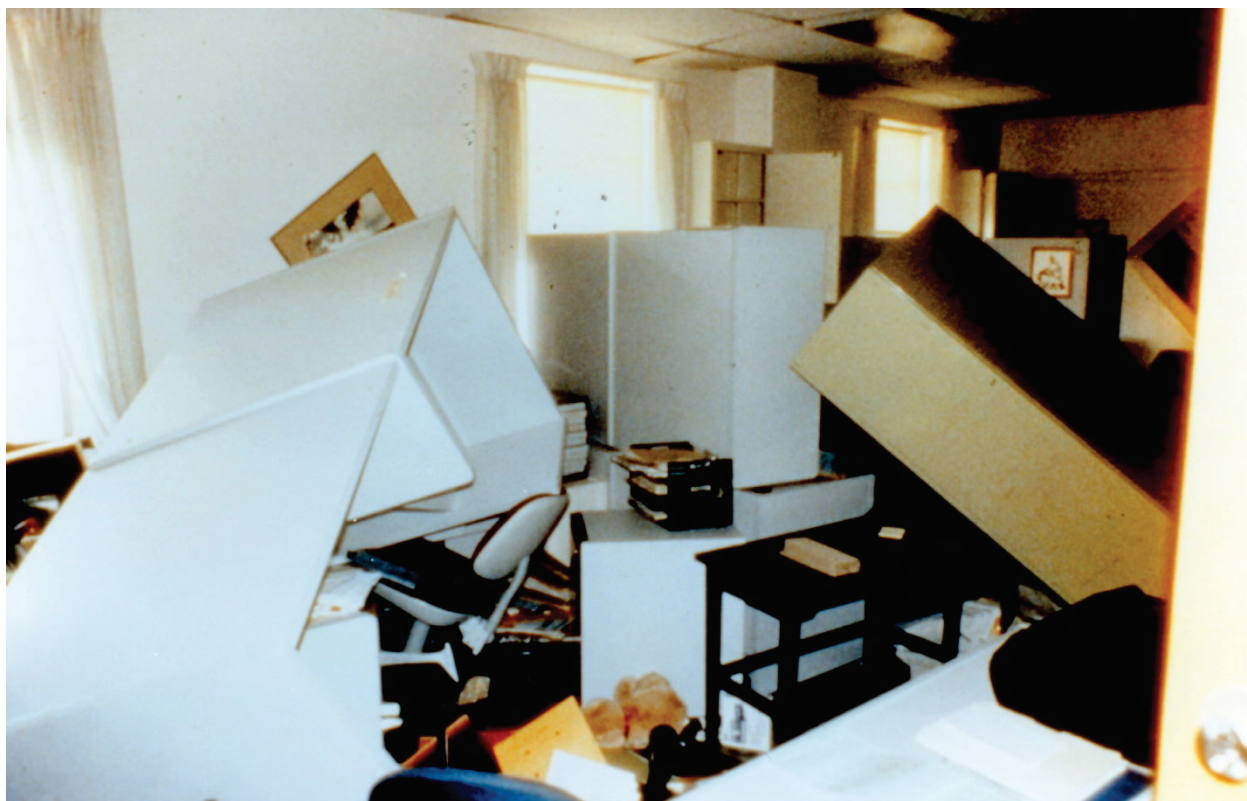
Figure 6.5.5.2-1 Damage to demountable partitions at the Veterans Administration Medical Center in Sepulveda as a result of the 1994 magnitude-6.7 Northridge Earthquake (Photo courtesy of James O. Malley).
