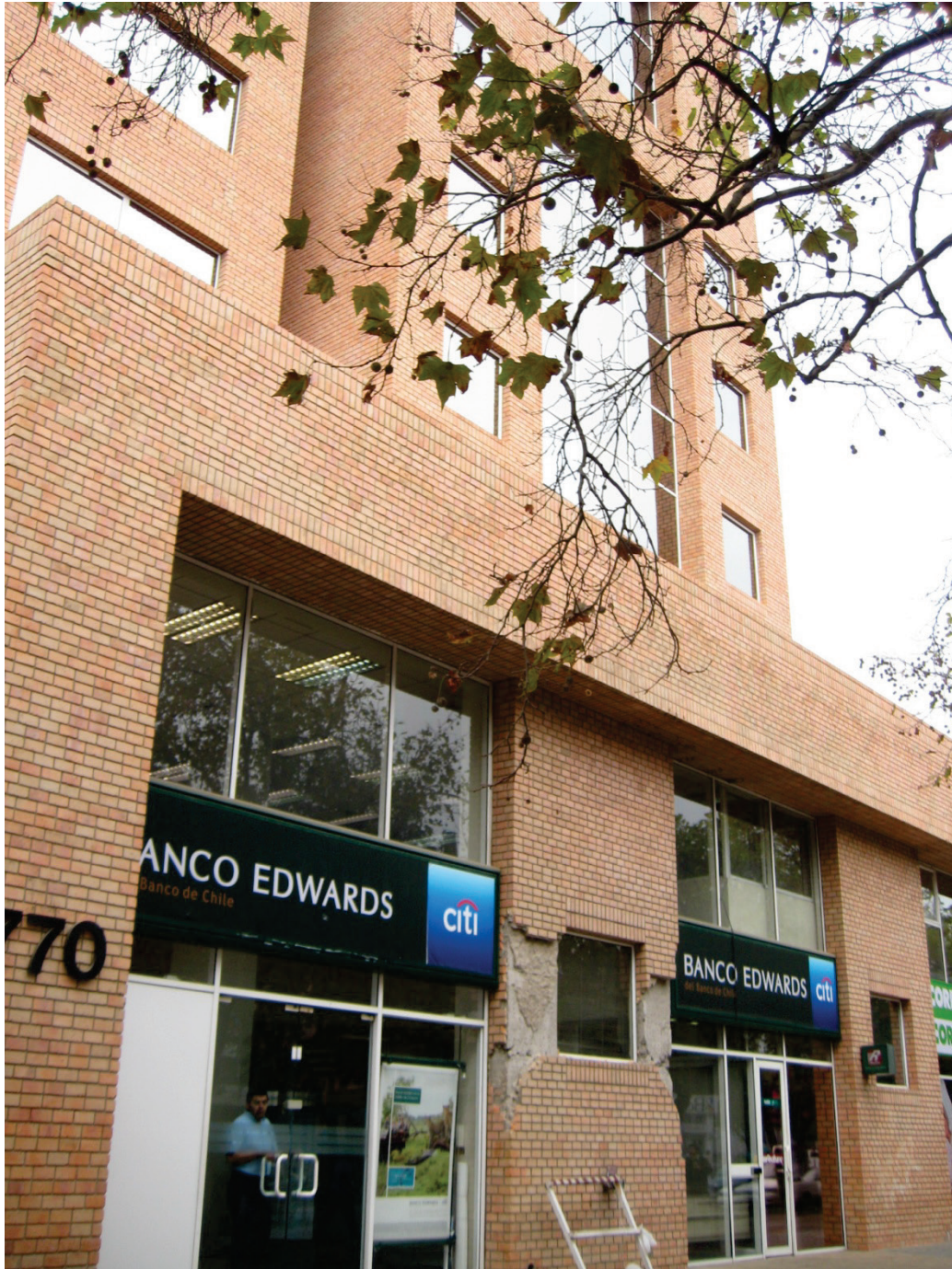
Figure 6.3.1.1-3 Cracked and spalled adhered veneer reveals incipient structural damage to concrete piers in Viña del Mar following the 2010 magnitude-8.8 Chile Earthquake. In this case, the areas of structural and nonstructural damage coincide; the adhered veneer remained intact over portions of the shear wall that did not deform significantly (Photo courtesy of Santiago Pujol, Purdue University).
