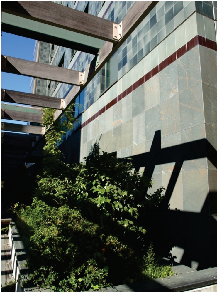
Figure 6.3.1.1-5 Landscaping strip restricts pedestrian access adjacent to adhered veneer façade. Larger units used within lower 6 feet; smaller units used above (Photo courtesy of Cynthia Perry, BFP Engineers).
