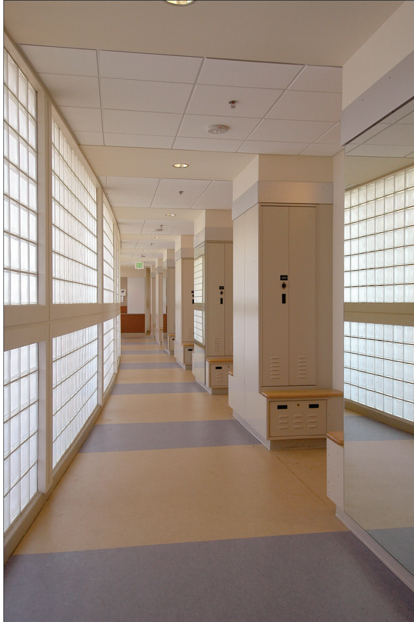
Figure 6.3.1.5-5 Glass block panels divided into numerous subpanels at the Chula Vista Police Headquarters, California (Photo courtesy of Pittsburgh Corning Corporation). In addition, the nonbearing glass block panel partition wall is isolated from seismic movement of the building structure.
