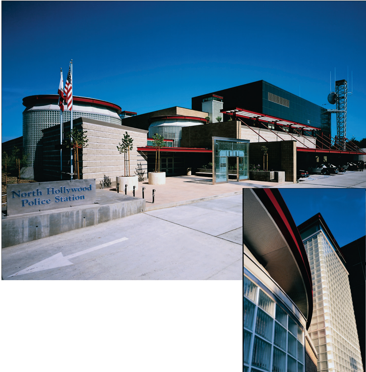
Figure 6.3.1.5-4 Use of glass block panels for select exterior and interior walls at the North Hollywood Police Station in California, utilizing standard details provided by Pittsburgh Corning Glass (Photo courtesy of Pittsburgh Corning Corporation).
