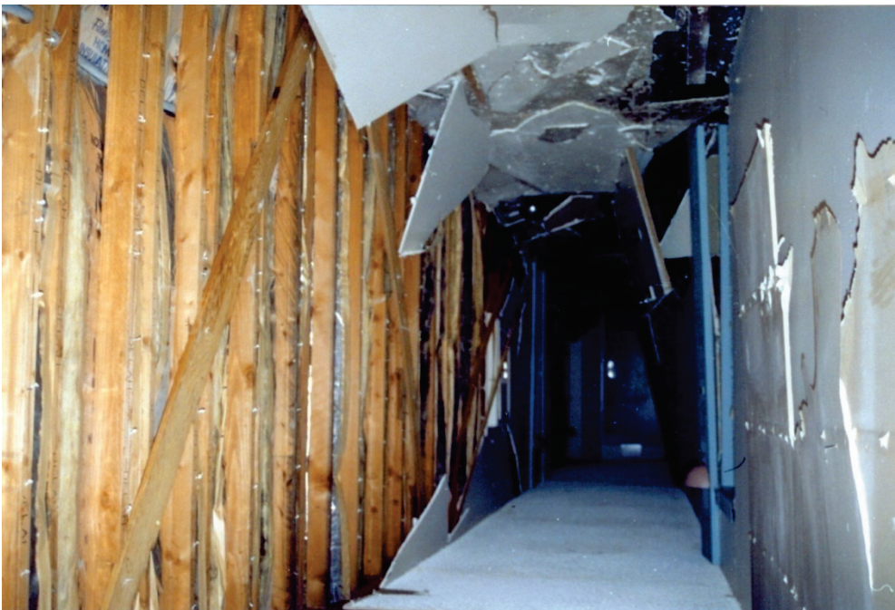
Figure 6.3.2.2-2 In-plane damage to wood stud wall spanning floor-to-floor caused by differential movement between the two floors in the 1994 Northridge Earthquake (Photo courtesy of Wiss, Janney, Elstner Associates).
