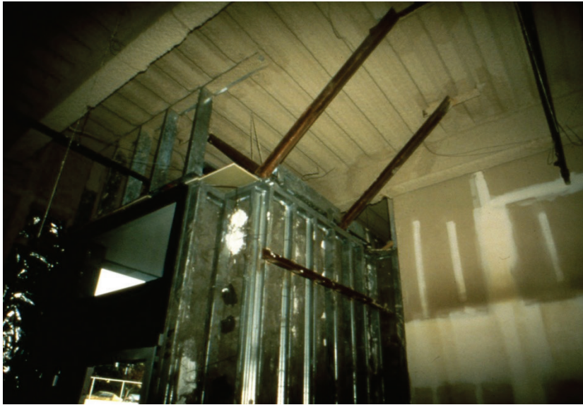
Figure 6.3.2.2-4 Bracing of partial height stud partition (Photo courtesy of Degenkolb Engineers).
