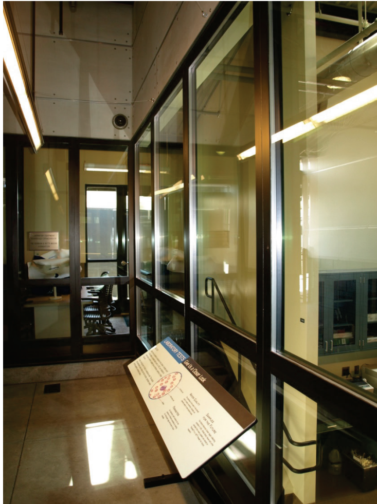
Figure 6.3.2.3-4 Glazed partition supported at base with slip track at top; partition above glazing suspended and braced from above. Glazing subdivided into relatively small panels with ample clearance at mullions (Photo courtesy of Cynthia Perry, BFP Engineers).
