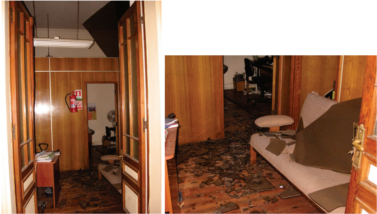
Figure 6.3.2.3-1 Glass shards fallen from the top of partial height office partitions in the reception area during the magnitude-8.8 2010 Chile Earthquake (Photo courtesy of Rodrigo Retamales, Rubén Boroscchek & Associates).
