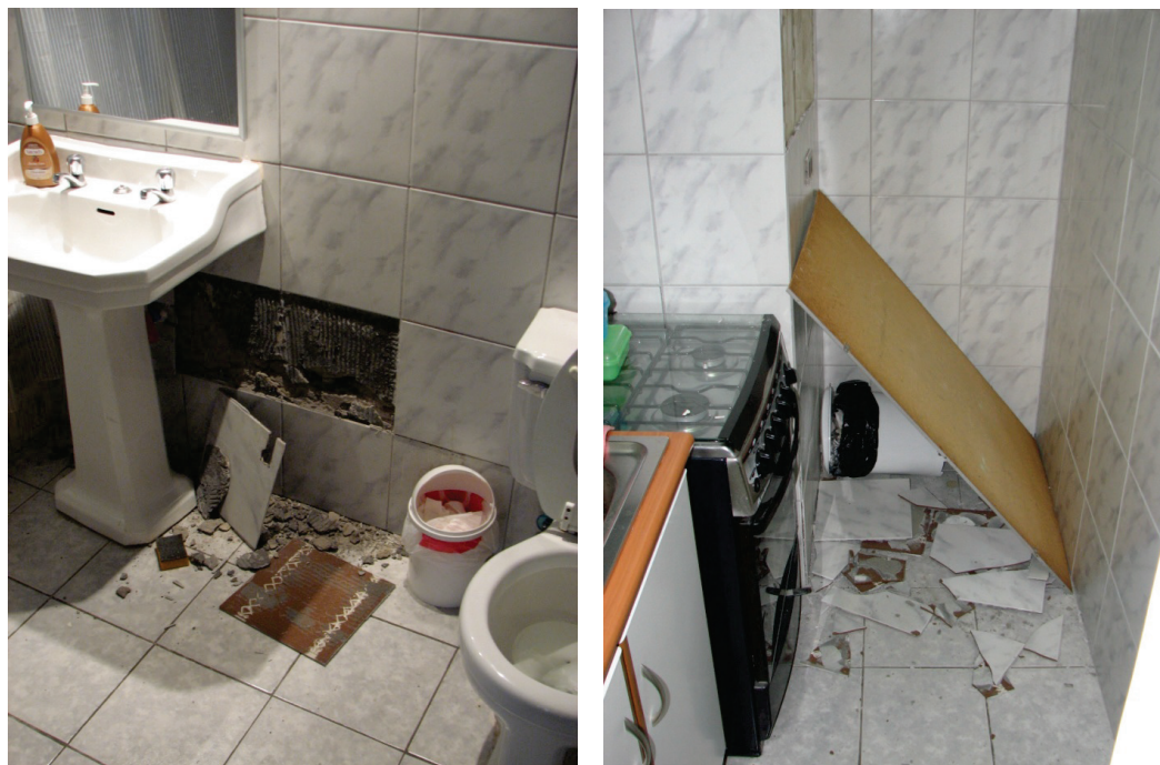
Figure 6.3.3.1-1 Damage to adhered tile veneer in residential bathroom and kitchen in the 2010 magnitude-8.8 Chile Earthquake (Photo courtesy of Antonio Iruretagoyena, Ruben Boroschek & Associates). Tile is adhered to CMU infill partitions.
