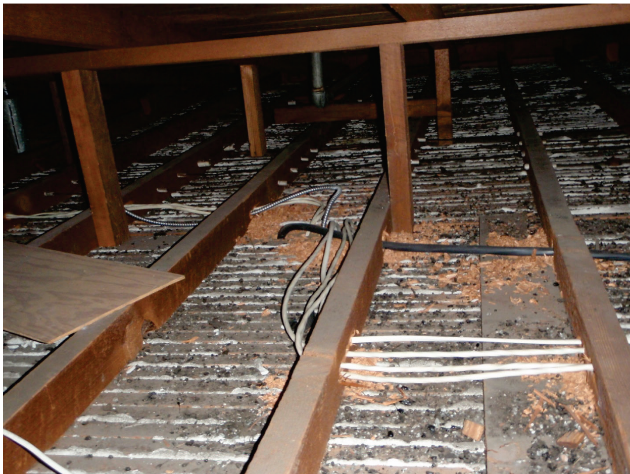
Figure 6.3.4.2-7 View of typical wood lath and plaster ceiling from the 1920's from above (Photo courtesy of Cynthia Perry, BFP Engineers). The wood lath is well nailed to the underside of the ceiling joists. This type of ceiling typically remains intact during an earthquake but may require crack repair and painting. Where the plaster has delaminated from the lath due to age or water leakage, wood strips could be installed from below as in Figure 6.3.4.2-8.
