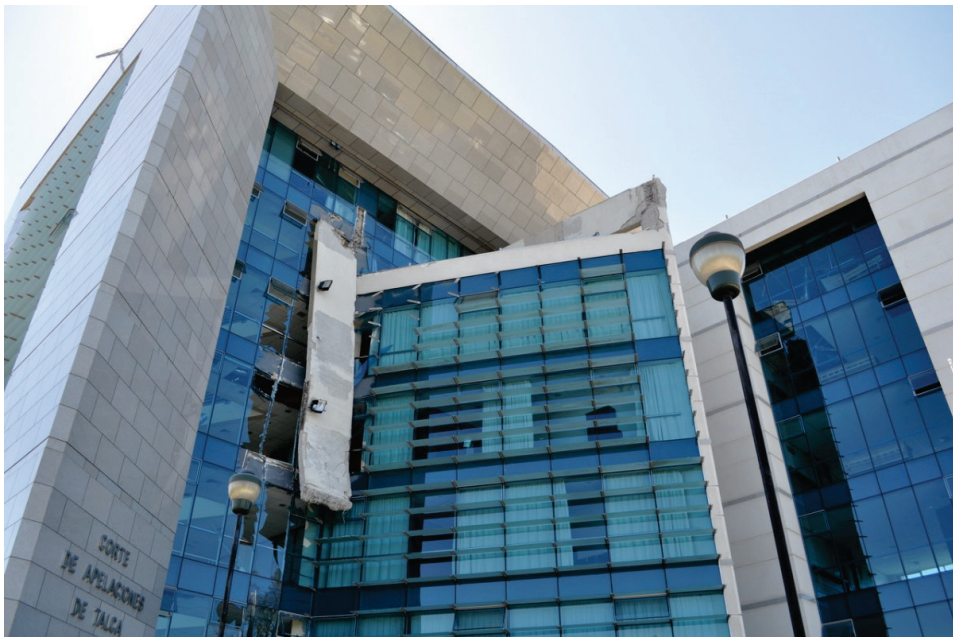
Figure 6.3.6.1-2 Reinforced concrete appendage dangling from connection on one side; impact damaged the curtain wall and created a serious hazard above the entrance of the Corte de Apelaciones de Talca in the 2010 magnitude-8.8 Chile Earthquake (Photo courtesy of Eduardo Fierro, BFP Engineers).
