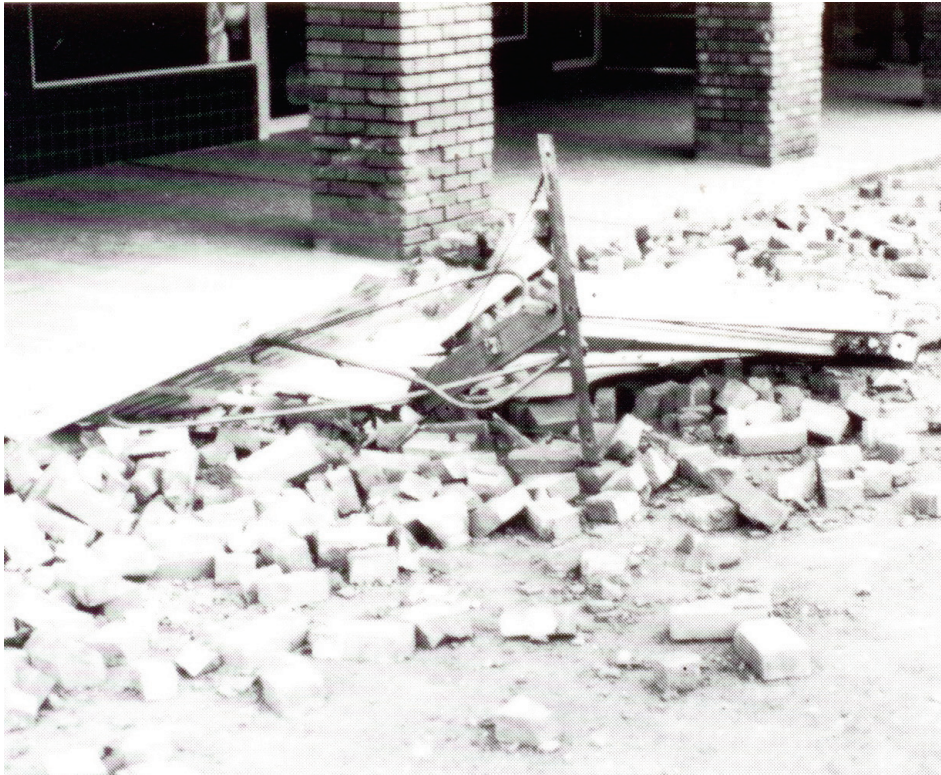
Figure 6.3.6.1-1 Failure of commercial sign in the 1979 Imperial Valley, California earthquake (Photo courtesy of Robert Reitherman).
