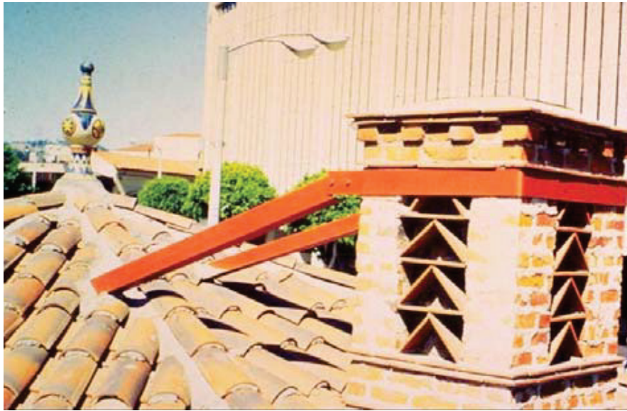
Figure 6.3.7.1-4 Braced chimney (FEMA, 2004).
