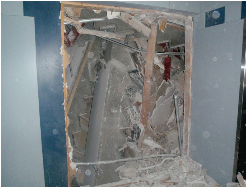
Figure 6.3.8.1-5 One story precast stair units stacked up at base of stairwell after falling off the sliding end supports and collapsing into stairwell (Photo courtesy of Des Bull, Holmes Consulting Group).
