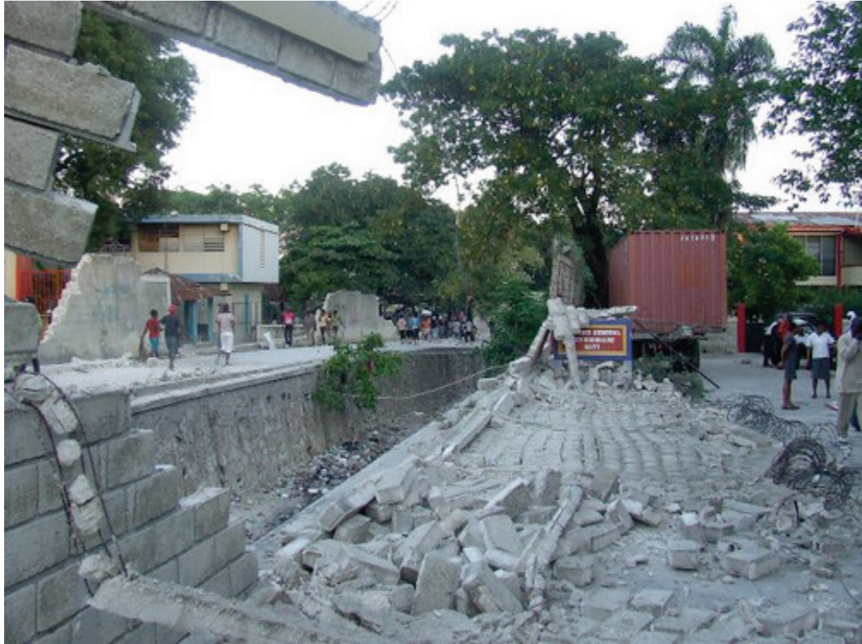
Figure 6.3.9.1-2 Freestanding masonry fences with inadequate reinforcement collapsed covering both sides of this street in Port-au-Prince in the 2010 magnitude-7 Haiti Earthquake (Photo courtesy of Yves Montoban). Many miles of such fencing collapsed in the 2010 Haiti Earthquake.
