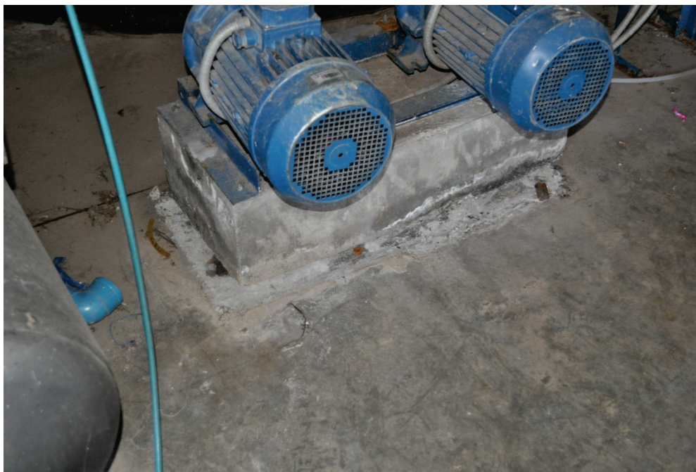
Figure 6.4.1.1-2 Pumps with rigid anchorage to housekeeping pad in the 2010 magnitude-8.8 Chile Earthquake; housekeeping pad not anchored to base slab and slid horizontally several inches (Photo courtesy of Eduardo Fierro, BFP Engineers).
