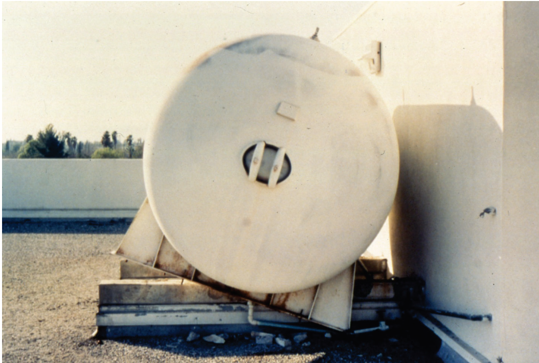
Figure 6.4.2.1-1 Tank shifted off support curb, Granada Hills Hospital in the 1994 magnitude-6.7 Northridge Earthquake (Photo courtesy of OSHPD).
