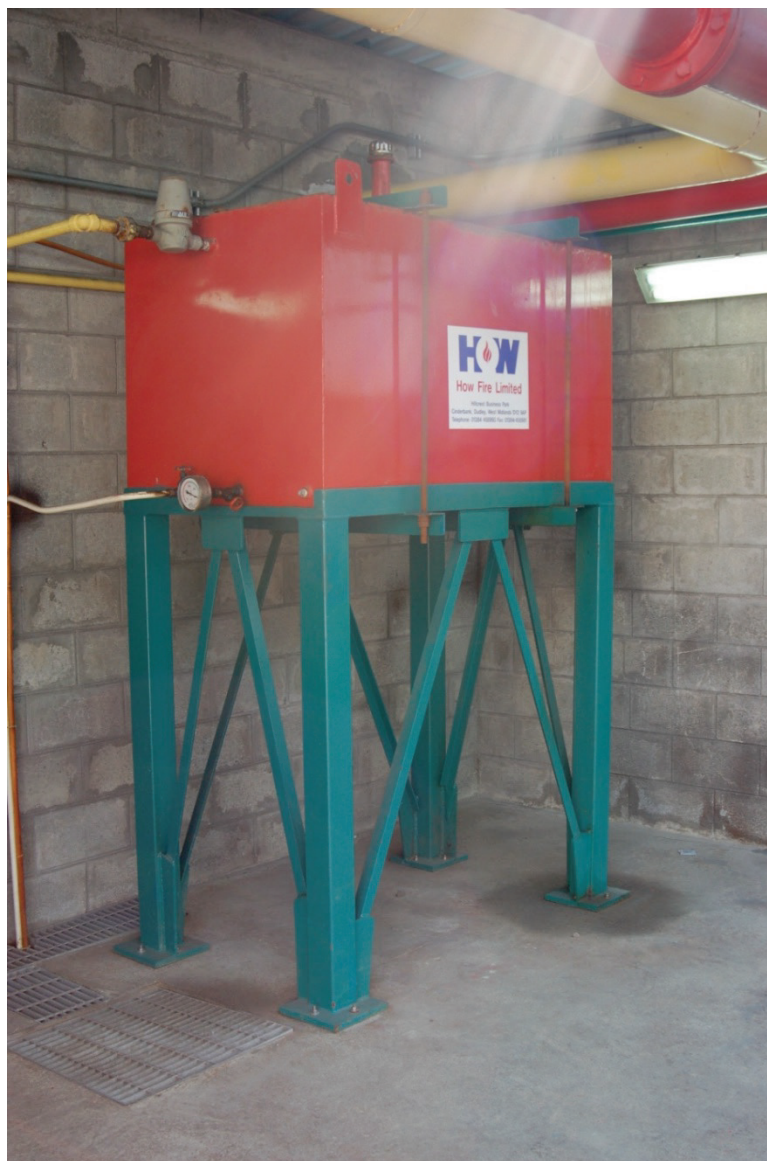
Figure 6.4.2.1-6 Braces added to four sides of tank support structure (Photo courtesy of Eduardo Fierro, BFP Engineers).
