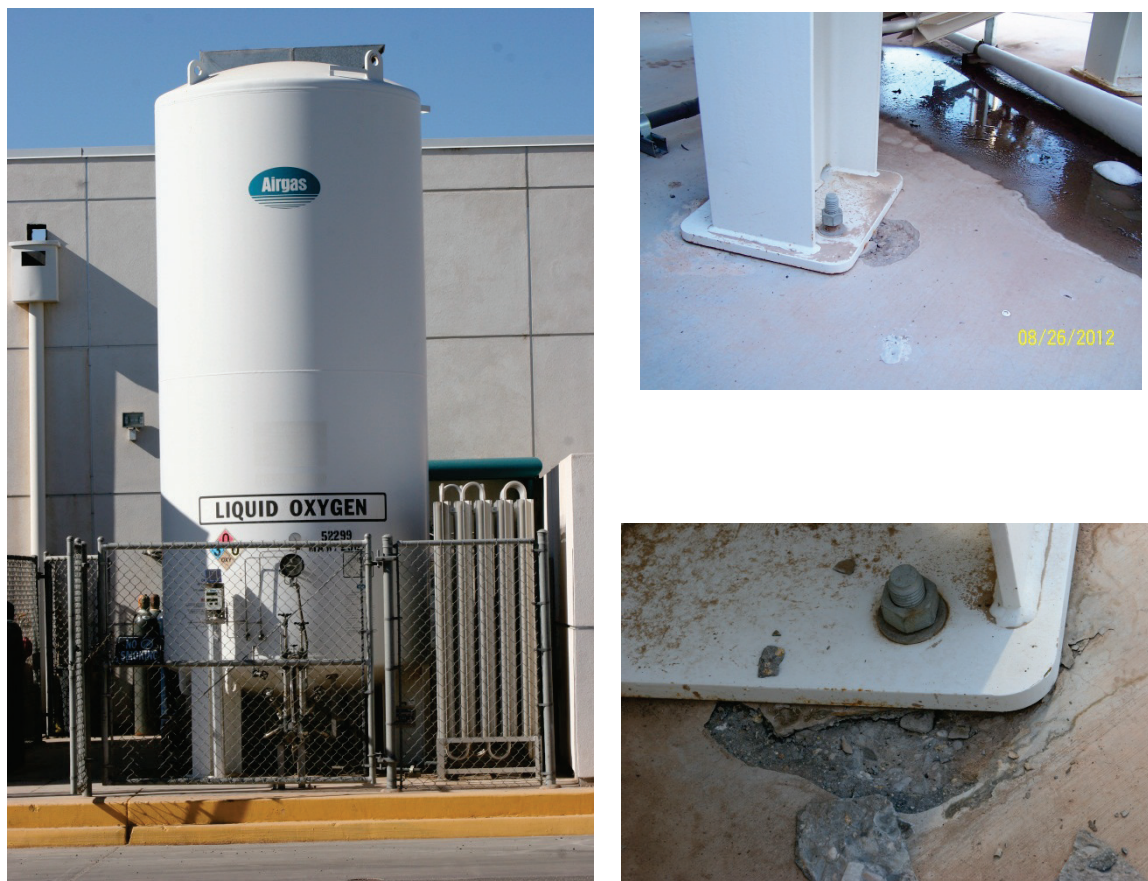
Figure 6.4.2.1-5 Damage to tanks at the Pioneer Memorial Hospital at the 2012 Brawley Earthquake (Photo courtesy of Chris Tokas, OSHPD)
