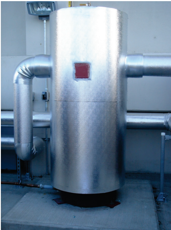
Figure 6.4.2.2-7 Examples of rigid base anchorage for small circular tanks (Photos courtesy of Maryann Phipps, Estructure).
