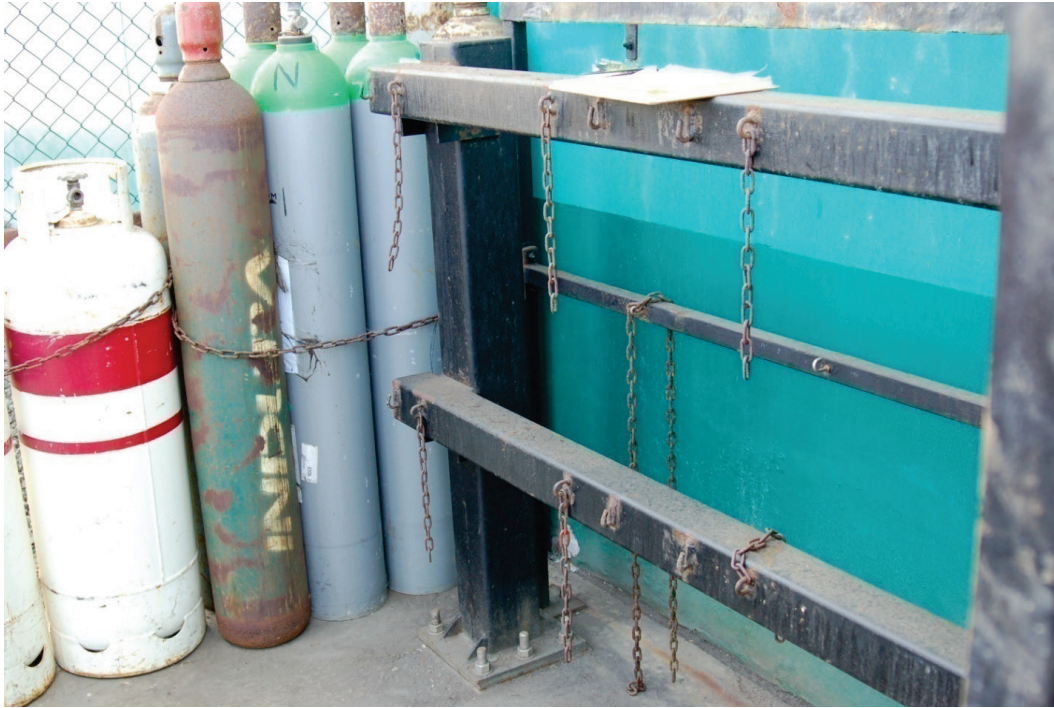
Figure 6.4.2.3-6 Detail of steel tube supports and chains (Photo courtesy of Eduardo Fierro, BFP Engineers).
