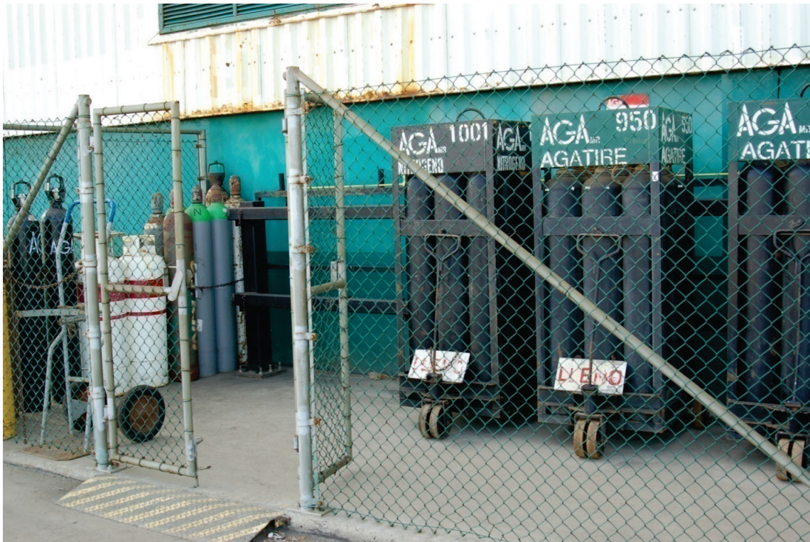
Figure 6.4.2.3-5 Steel tube supports for mobile gas cylinder carts (Photo courtesy of Eduardo Fierro, BFP Engineers).
