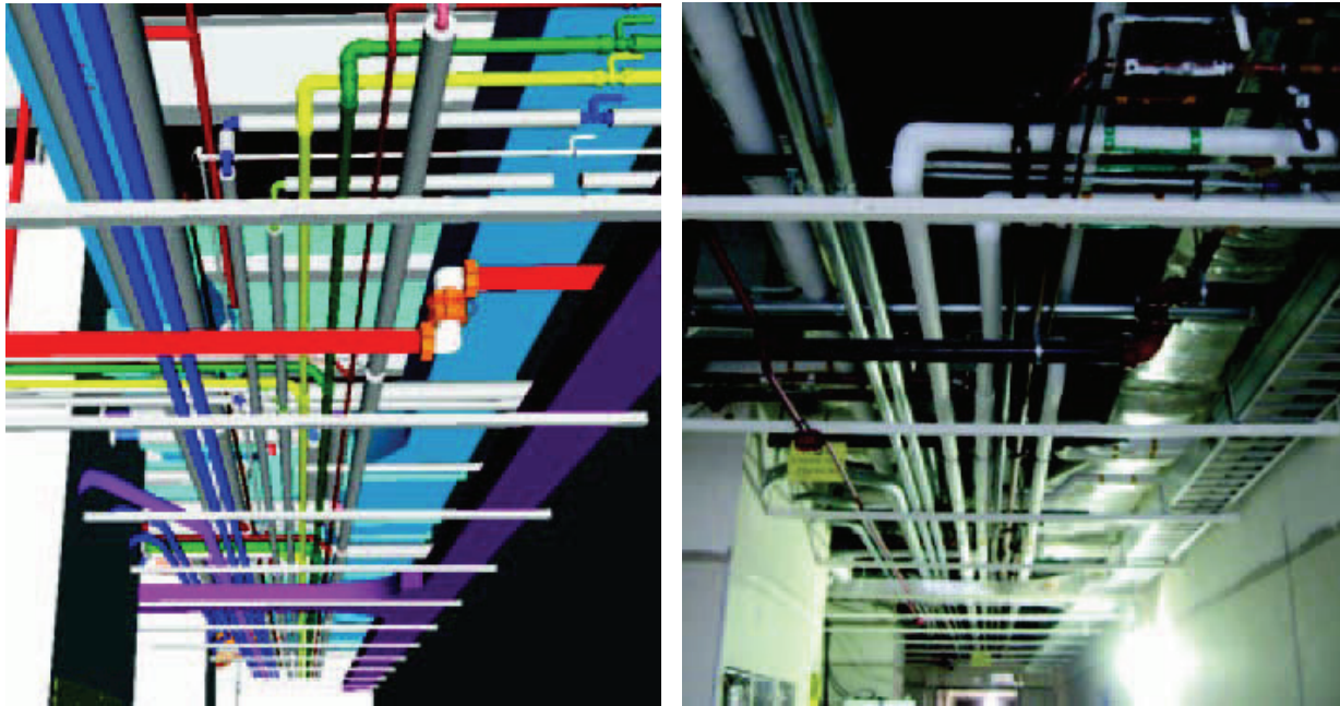
Figure 6.4.3.1-9 Example of BIM Model (left) compared to installed piping (right) (Photo and image courtesy of ISAT).
