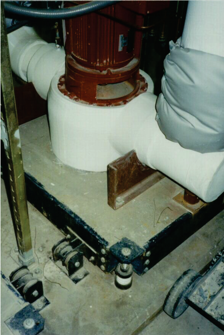
Figure 6.4.3.2-1 In-line pump mounted on independent concrete inertia pad with vibration isolation and seismic snubbers (Photo courtesy of Mason Industries).
