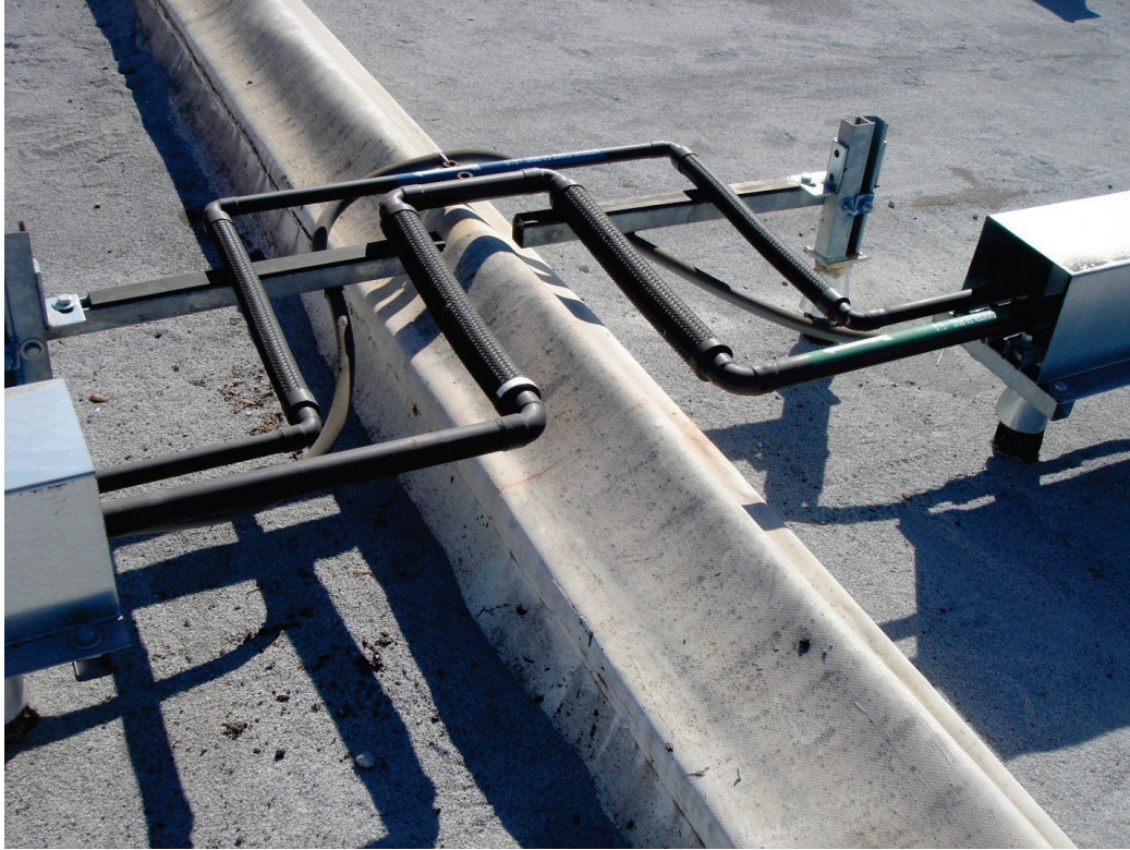
Figure 6.4.3.3-4 Flexible pipe connections at rooftop expansion joint (Photo courtesy of Maryann Phipps, Estructure).
