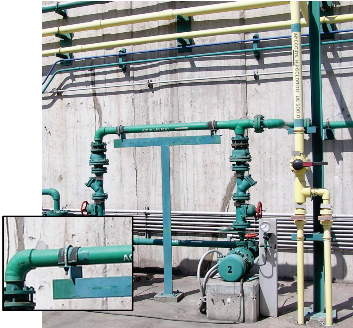
Figure 6.4.3.5-1 Pipe and support assembly seem intact but photo shows evidence of longitudinal movement of the pipe in the U-bolts (Photo courtesy of BFP Engineers). A rubber pad was installed between the U-bolt and pipe in order to increase the friction coefficient, but was not sufficient to provide longitudinal restraint.
