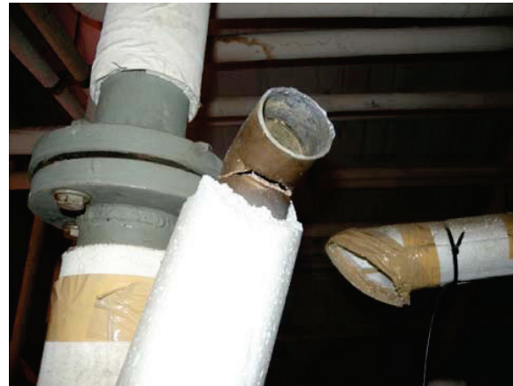
Figure 6.4.5.2-1 Broken copper hot water piping for at the San Carlos Hospital in the 2010 Chile Earthquake. Piping failure caused by movement of inadequately braced boiler shown at left (Photos courtesy of Gilberto Mosqueda, SUNY Buffalo).
