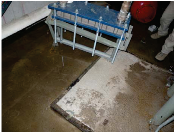
Figure 6.4.5.2-1 Broken copper hot water piping for at the San Carlos Hospital in the 2010 Chile Earthquake. Piping failure caused by movement of inadequately braced boiler shown at left (Photos courtesy of Gilberto Mosqueda, SUNY Buffalo).
