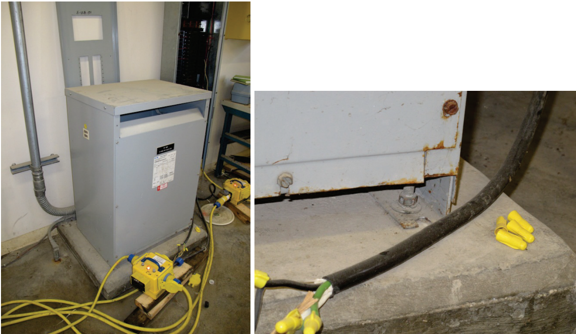
Figure 6.4.7.3-2 Typical electrical distribution dry type transformer. Note the use of manufacturer supplied anchor locations on base channels. Post earthquake photo from the 2010 Haiti M 7.0 Earthquake (photos courtesy of Philip J. Caldwell).
