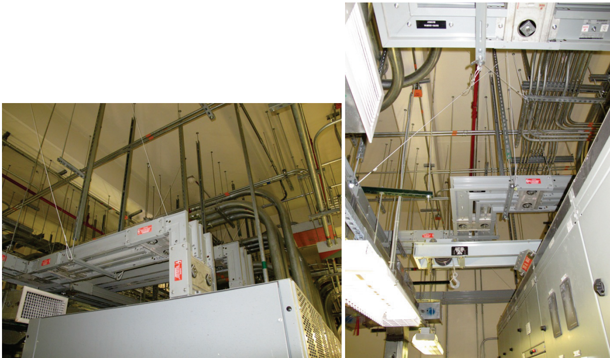
Figure 6.4.7.3-3 High ampacity power busway routing power from generator paralleling switchgear to facility. Note use of lateral restraints in addition to gravity hanger. Supplied uninterrupted power to critical facility during the 2010 M 7.0 Haiti earthquake. (photos courtesy of Philip J. Caldwell)
