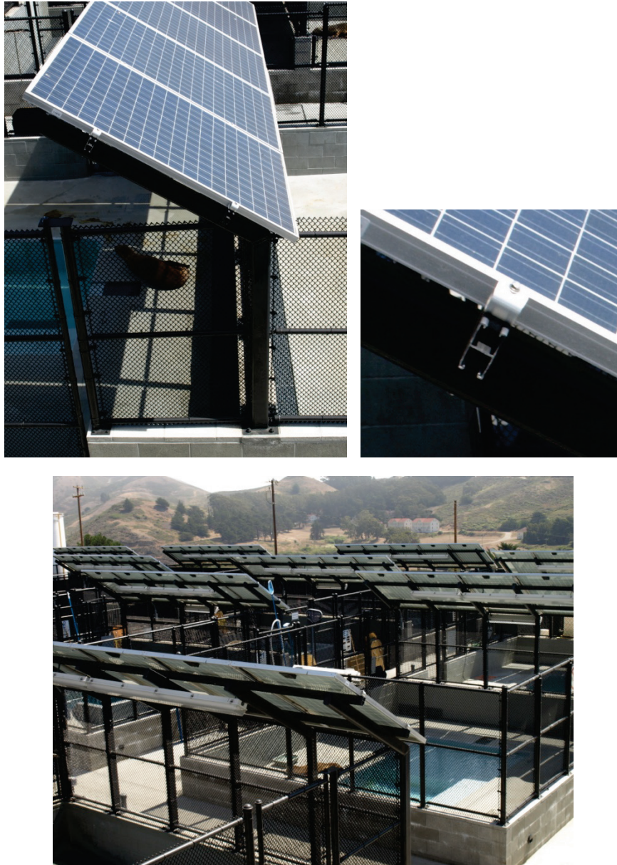
Figure 6.4.7.5-2 Ground mounted photovoltaic system that also provides shade to injured animals at the Marine Mammal Center in Sausalito, California (Photo courtesy of Cynthia Perry, BFP Engineers). Each solar panel is screwed to the strut at four locations; two rows of struts are bolted to 6 steel tubes which are anchored at the base with four bolts apiece.
