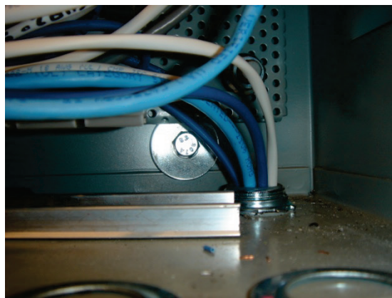
Figure 6.4.8.2-2 Wall anchorage for electrical panel; standard strut anchored to wall studs and panel anchored to strut (Photo courtesy of Maryann Phipps, Estructure).
