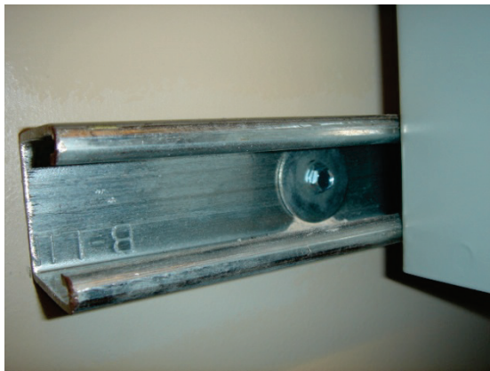
Figure 6.4.8.2-2 Wall anchorage for electrical panel; standard strut anchored to wall studs and panel anchored to strut (Photo courtesy of Maryann Phipps, Estructure).
