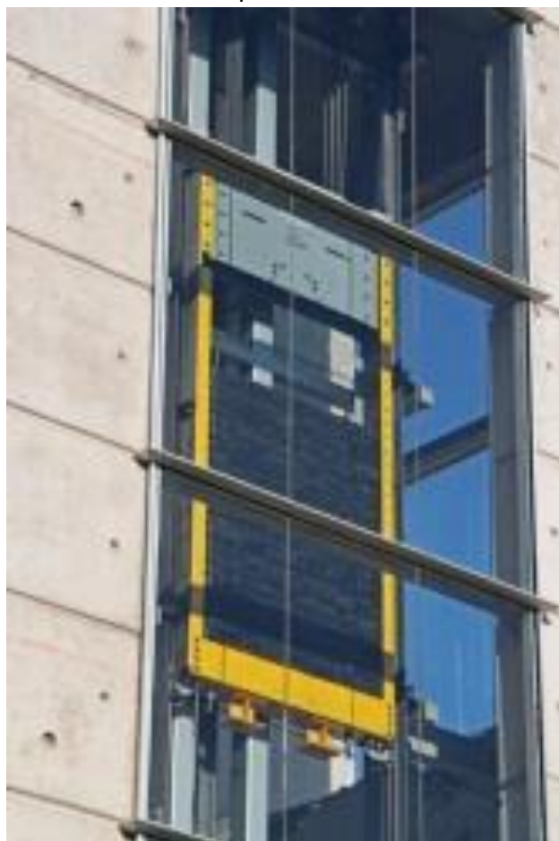
Figure 6.4.10.2-1 Examples of an elevator counterweight (Photo courtesy of Eduardo Miranda, Stanford University).
