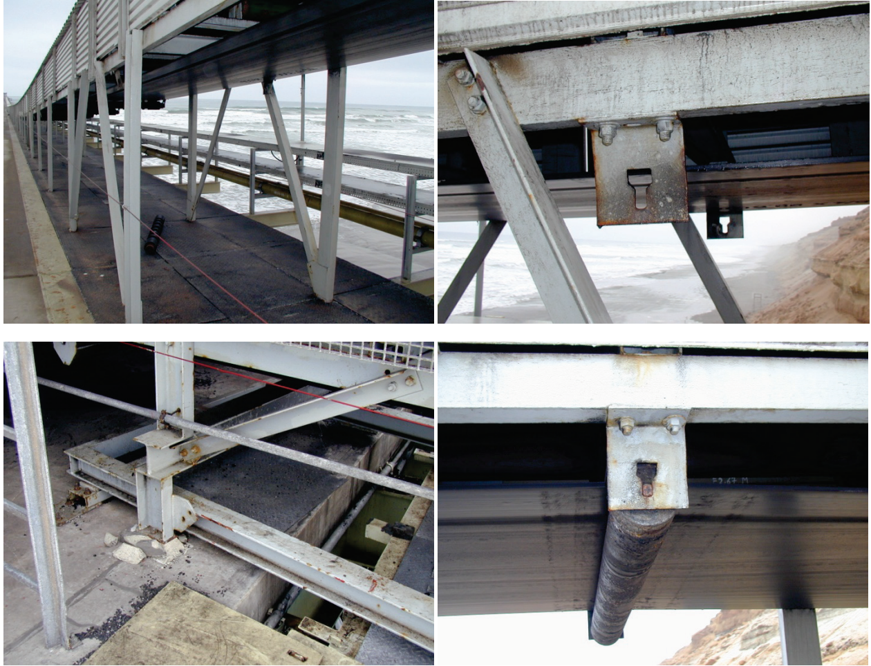
Figure 6.4.11.1-3 Damage to industrial coal conveyor on jetty in southern Peru in the 2001 magnitude-8.4 Peru Earthquake (Photos courtesy of Eduardo Fierro, BFP Engineers). Conveyor was well anchored along entire length but detailing at the seismic joint between the jetty and platform did not allow sufficient movement, resulting in misalignment at end of conveyor and damage to the supports as shown at lower left. Approximately 10% of the rollers fell; these were held in place with friction fittings and did not have positive connections.
