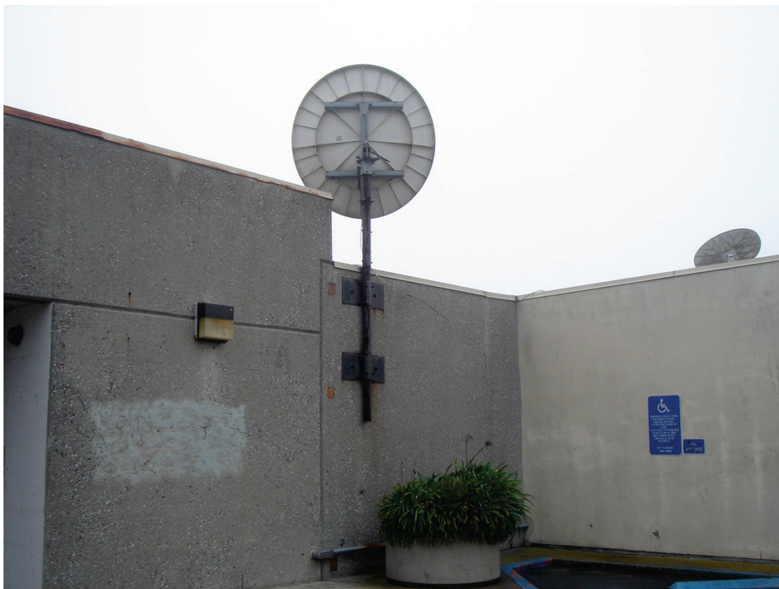
Figure 6.4.7.6-5 Antenna mast mounted to concrete wall surface at top floor of building (Photo courtesy of (Photo courtesy of Maryann Phipps, Estructure). Note that two wall brackets are used to resist moments produced by wind or seismic forces. This antenna is larger than most standard residential versions.
