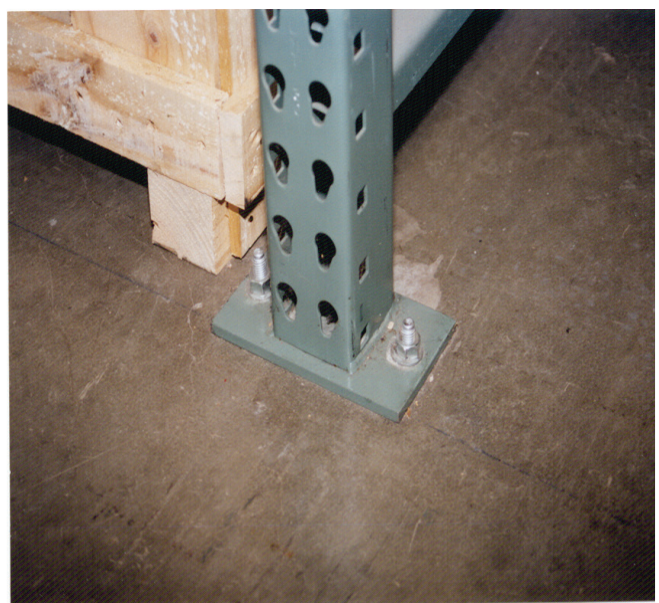
Figure 6.5.1.2-5 Typical pallet storage rack configuration and details (Photos courtesy of Maryann Phipps, Estructure).
