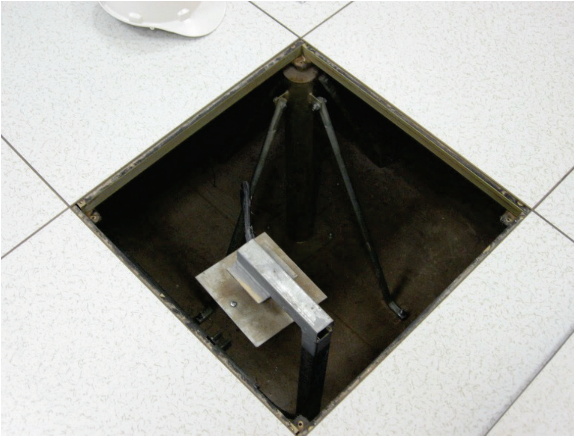
Figure 6.5.3.1-3 Undamaged access floor with braced pedestals in the 2010 Chile Earthquake (Photo courtesy of Rodrigo Retamales, Rubén Boroschek & Associates).
