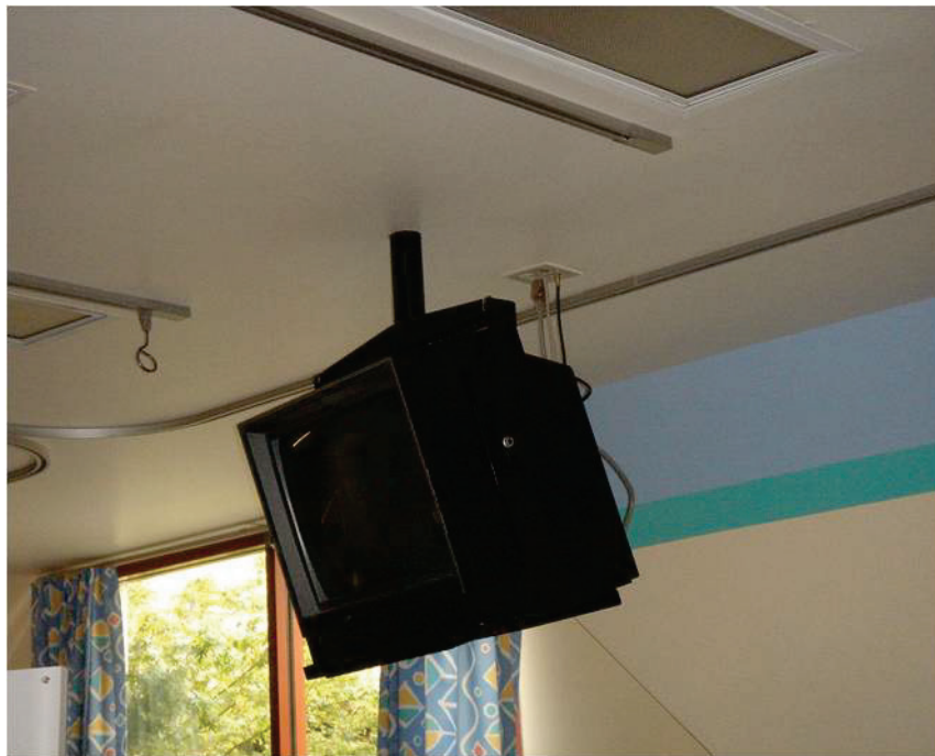
Figure 6.5.3.4-3 Mounting plate above ceiling for overhead television bracket in a hospital room. Television or monitor must be securely attached to the bracket (Photos courtesy of Maryann Phipps, Estructure).
