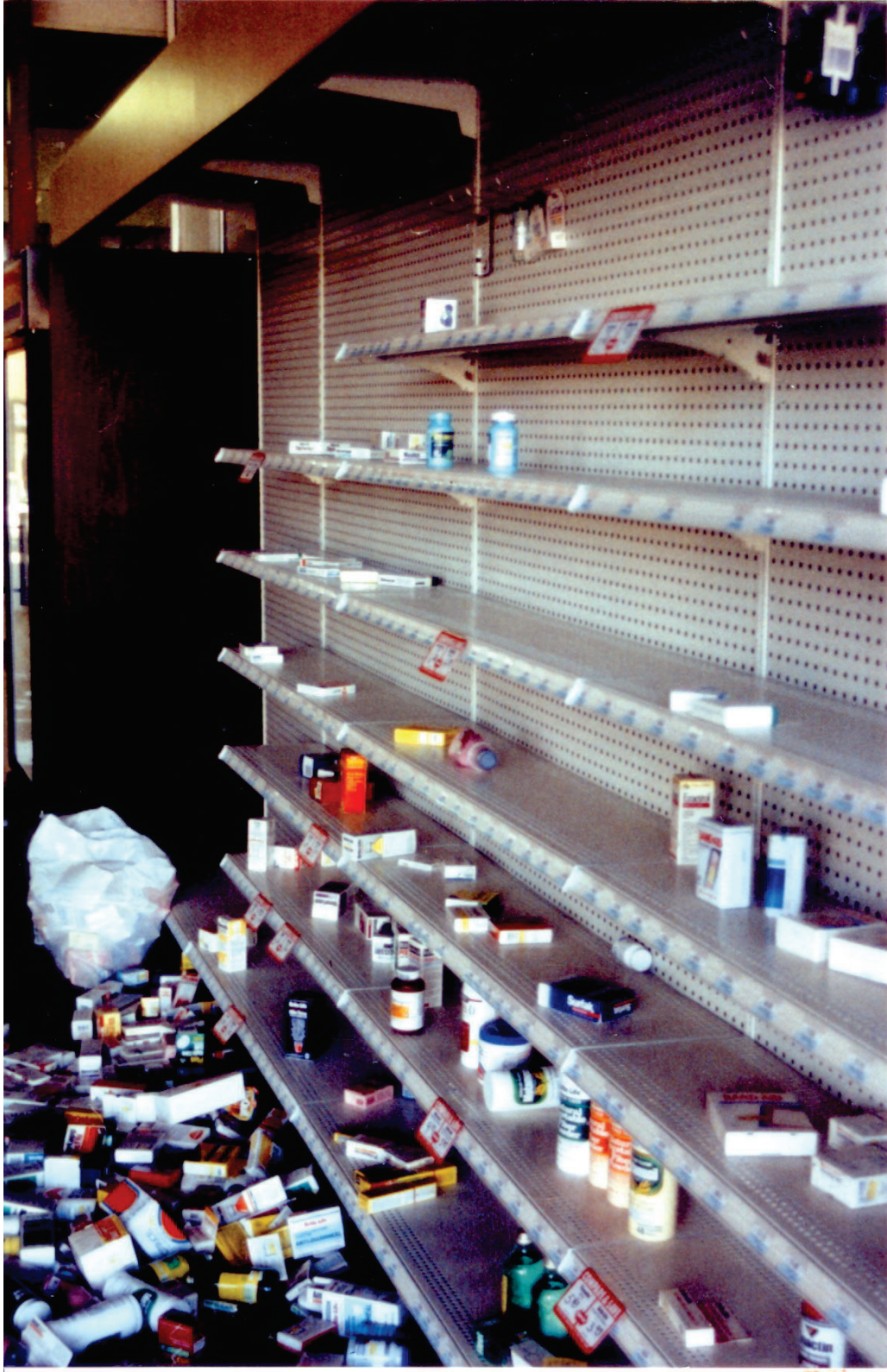
Figure 6.5.4.1-2 Spilled pharmaceutical and medical supplies in the 1994 magnitude-6.7 Northridge Earthquake (Photo courtesy of Robert Reitherman).
