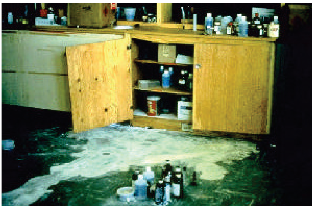
Figure 6.5.4.1-1 Spilled chemicals in high school chemistry lab in the 1971 magnitude-6.6 San Fernando Earthquake (Photo courtesy of EERI).
