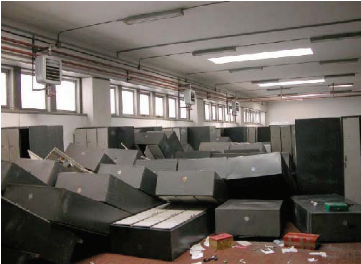
Figure 6.5.5.1-3 Unanchored cabinets toppled in the 1994 Northridge Earthquake (Photo courtesy of Wiss, Janney, Elstner)
