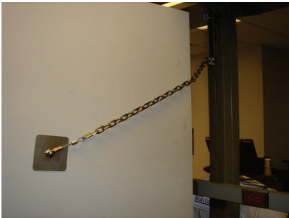
Figure 6.5.5.3-5 Typical tethering details for kitchen equipment and vending machines. Tether provided on both sides of equipment and does not penetrate the equipment housing (Photos courtesy of Maryann Phipps, Estructure).
