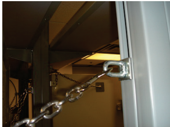
Figure 6.5.5.3-5 Typical tethering details for kitchen equipment and vending machines. Tether provided on both sides of equipment and does not penetrate the equipment housing (Photos courtesy of Maryann Phipps, Estructure).
