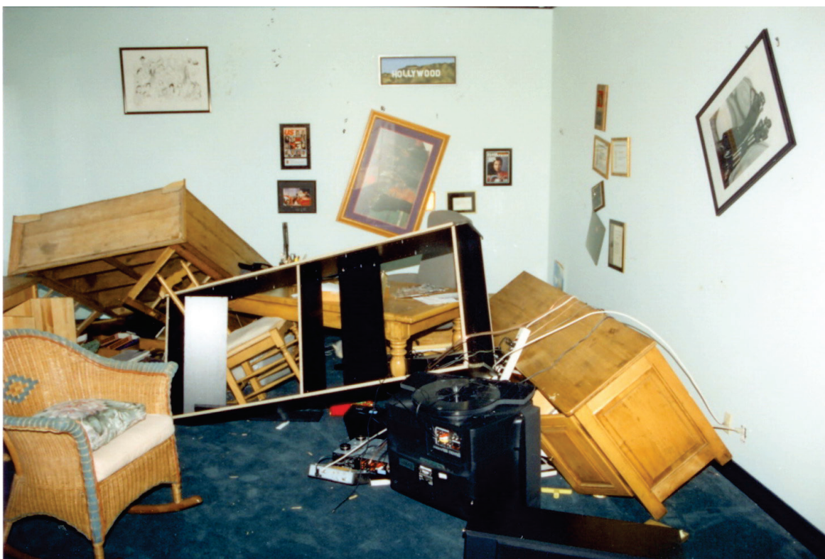
Figure 6.5.5.3-1 Residential damage in the 1994 magnitude-6.7 Northridge Earthquake (Photo courtesy of Wiss, Janney, Elstner Associates).
