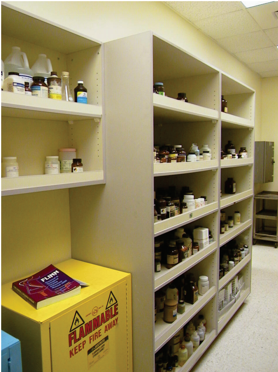
Figure 6.5.6.1-3 High school lab supplies protected on shelving with edge restraints (Photo courtesy of EQE for the Salt Lake City School District).
