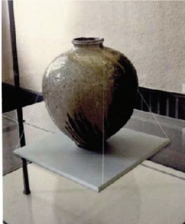
Figure 6.5.6.3-4 Seismic restraint of an object with artistic and historical value with nylon filament (fishing line) in the Tokyo Museum in Ueno Park (Photo courtesy of Robert Reitherman, CUREE).
